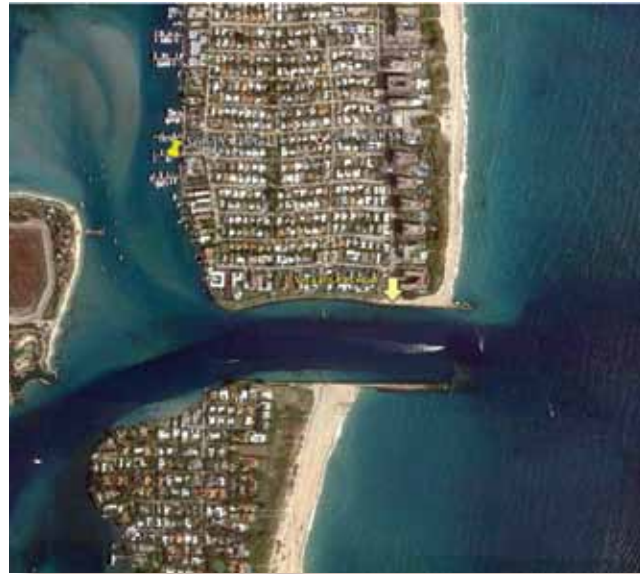
The indented south side of Lake Worth Inlet and the accumulation of sand inside the lagoon off Sailfish Marina are easily visible in this Google Earth image. Commercial inlets like this one must be periodically dredged to maintain safe navigation, however maintaining the inlet disrupts littoral drift.
